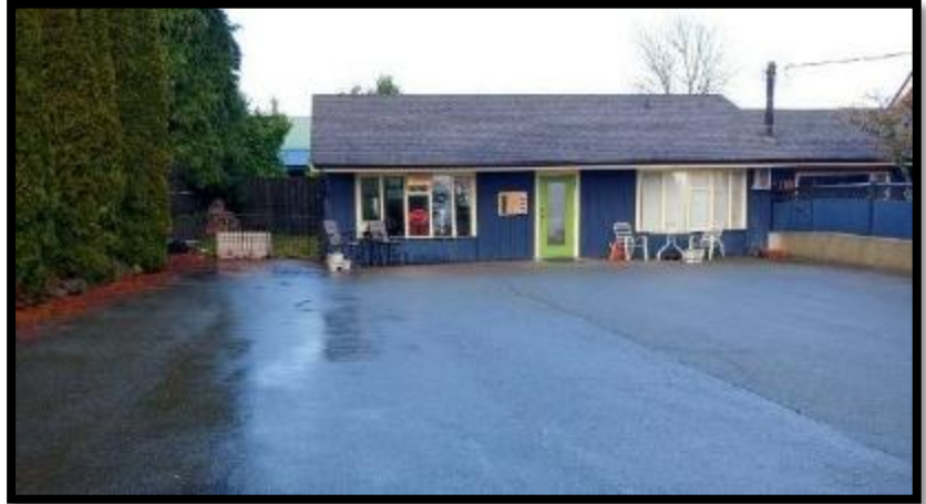
Figure 2: Existing front commercial façade at 204 Dogwood Drive.
