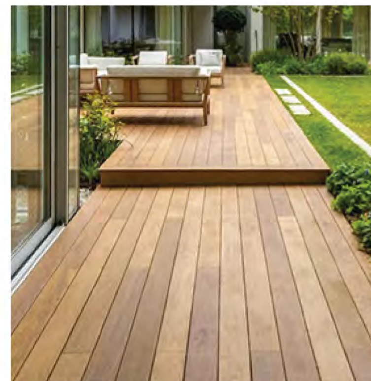
Verandah wood decking. Picture framed end boards to protect the end grain of decking. Clear finish
