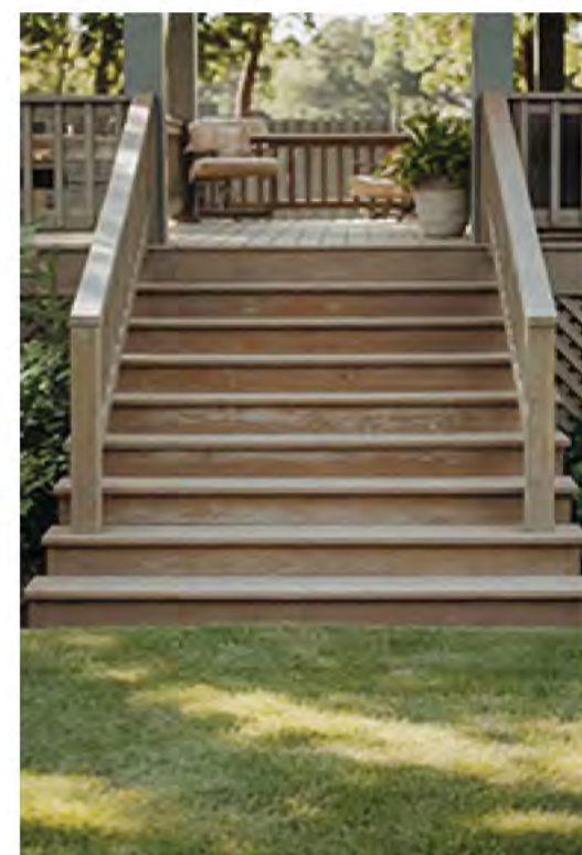
Wood stairs from grade to entry porches and decks. Clear seal finish
