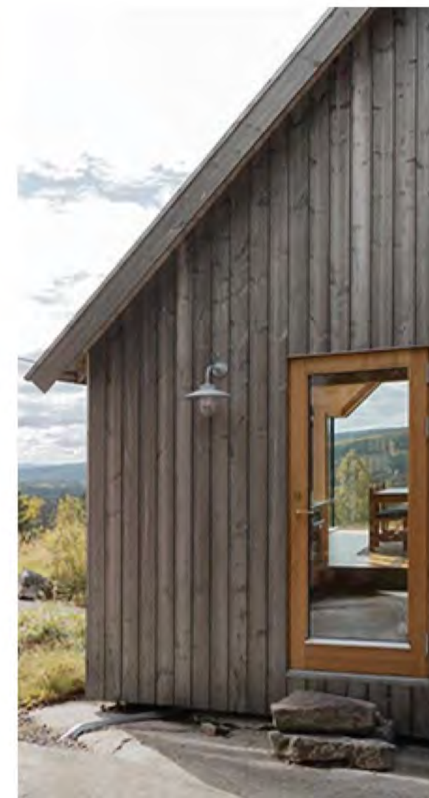
Vertical wood cladding. Glazed door with subtle lighting to mark the entry. Clear finish
