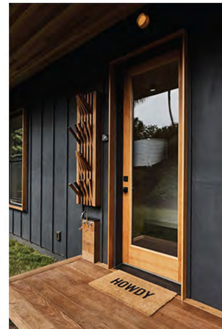
Entry porch with glazed door and subtle light to mark the entry. Clear finish
