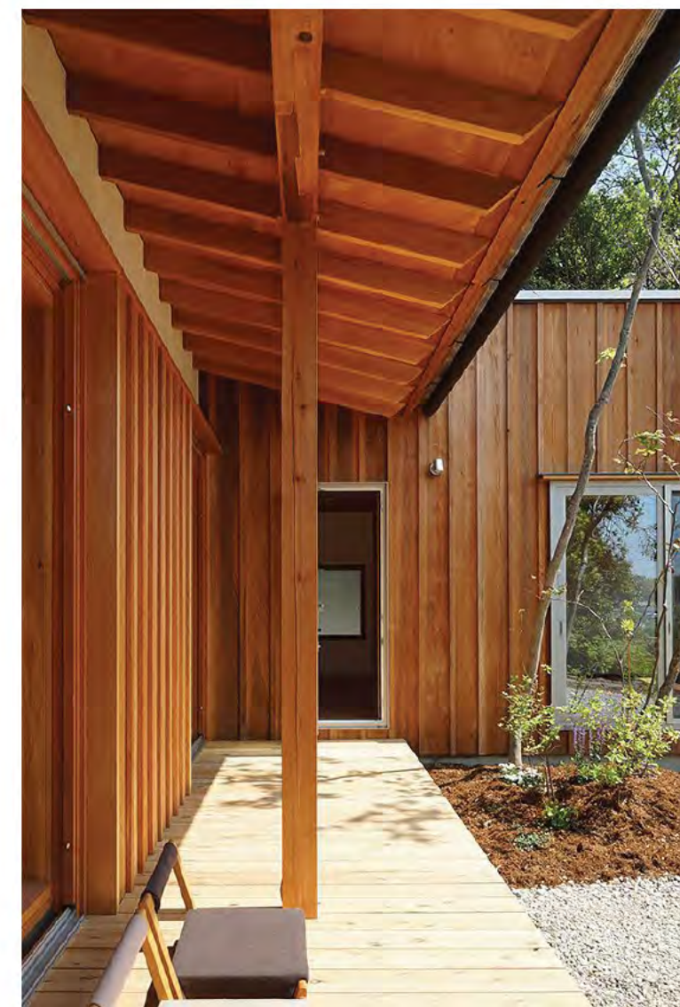
Exterior verandah exposed wood posts, beams and rafters. Clear finish
