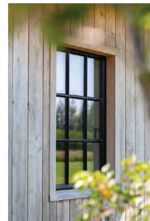
Black window frame in vertical wood cladding. Window trim to match cladding. Clear finish
