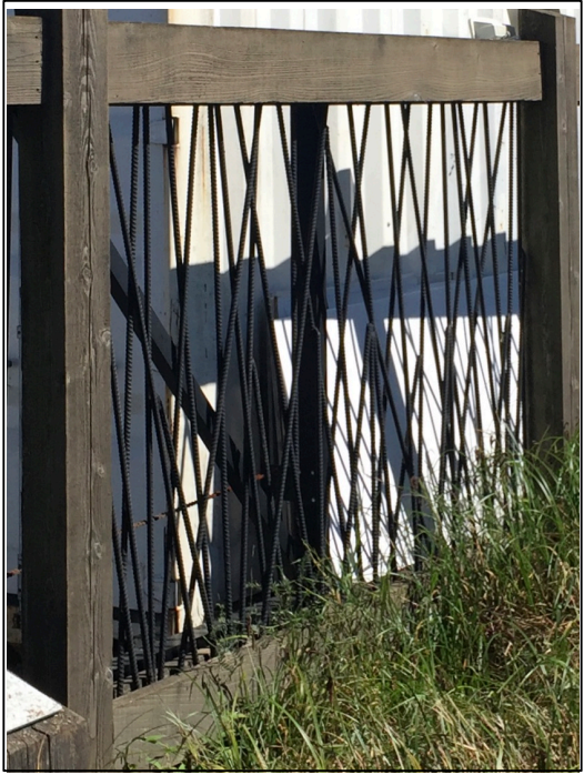
Patio enclosure design – wood frame with black metal pickets.
