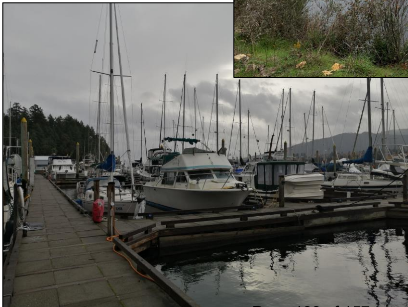
Photo 7: Looking SE along Dock A showing part of existing marina.
