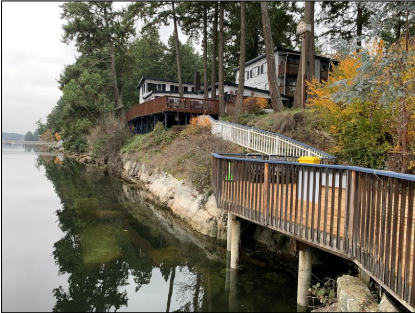
Photo 5: Looking NW at the Raven Point Inn and shoreline from the existing gangway.
