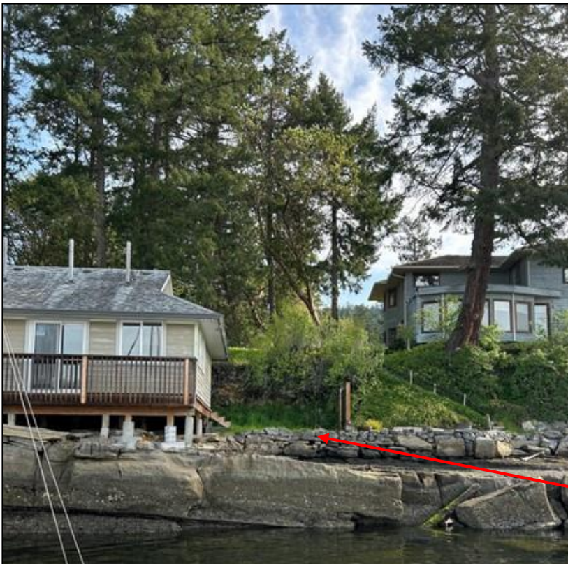
Photo 4: Photo provided by Cascara showing location for proposed new abutment, bridge, pier and gangway.
