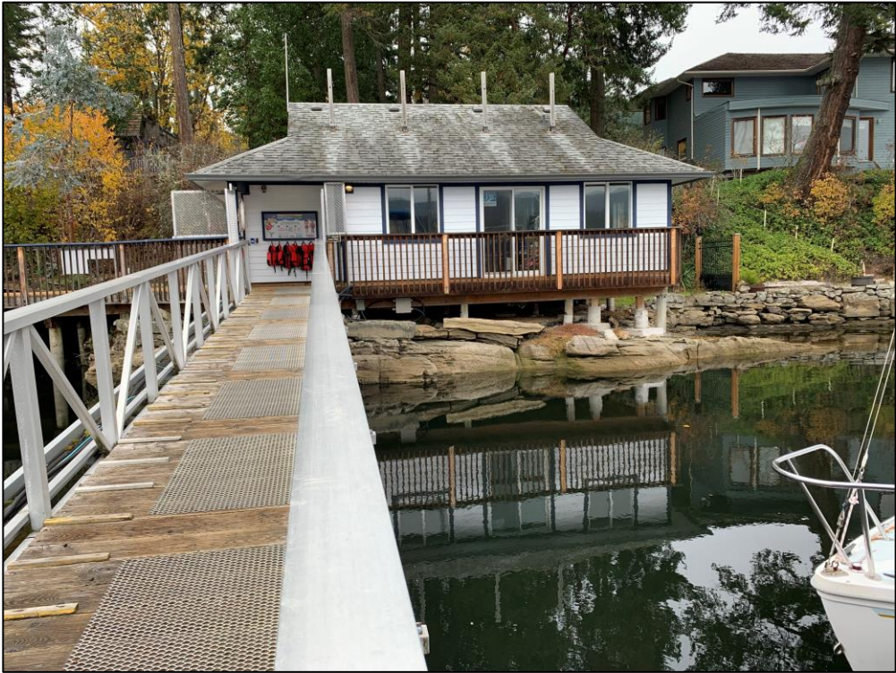
Photo 3: Showing the existing marina office from the end of the gangway looking NE.
