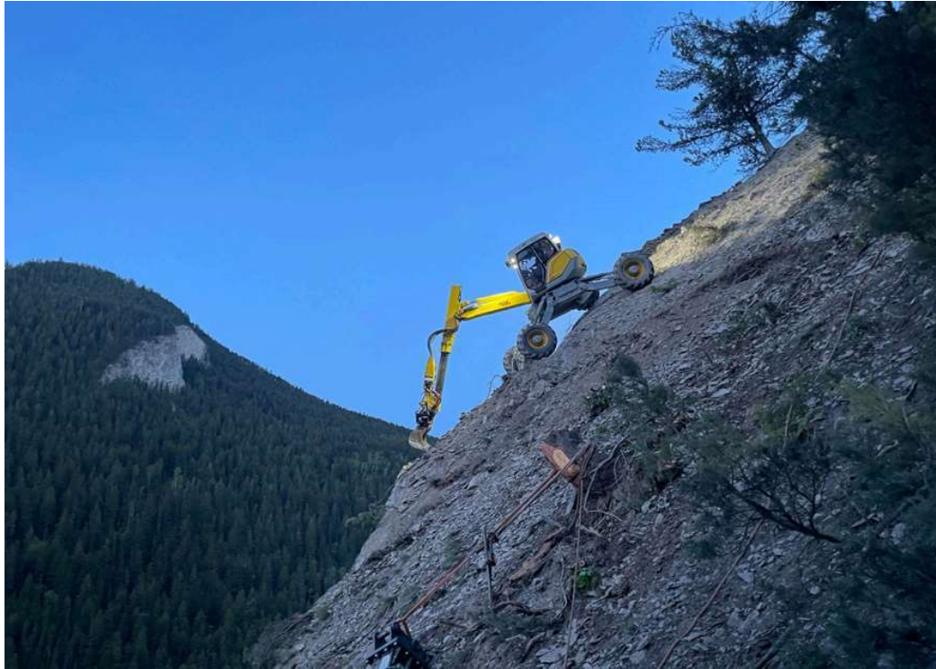
Photo 1 - Spider Excavator on 45° slope in Kicking Horse Canyon
