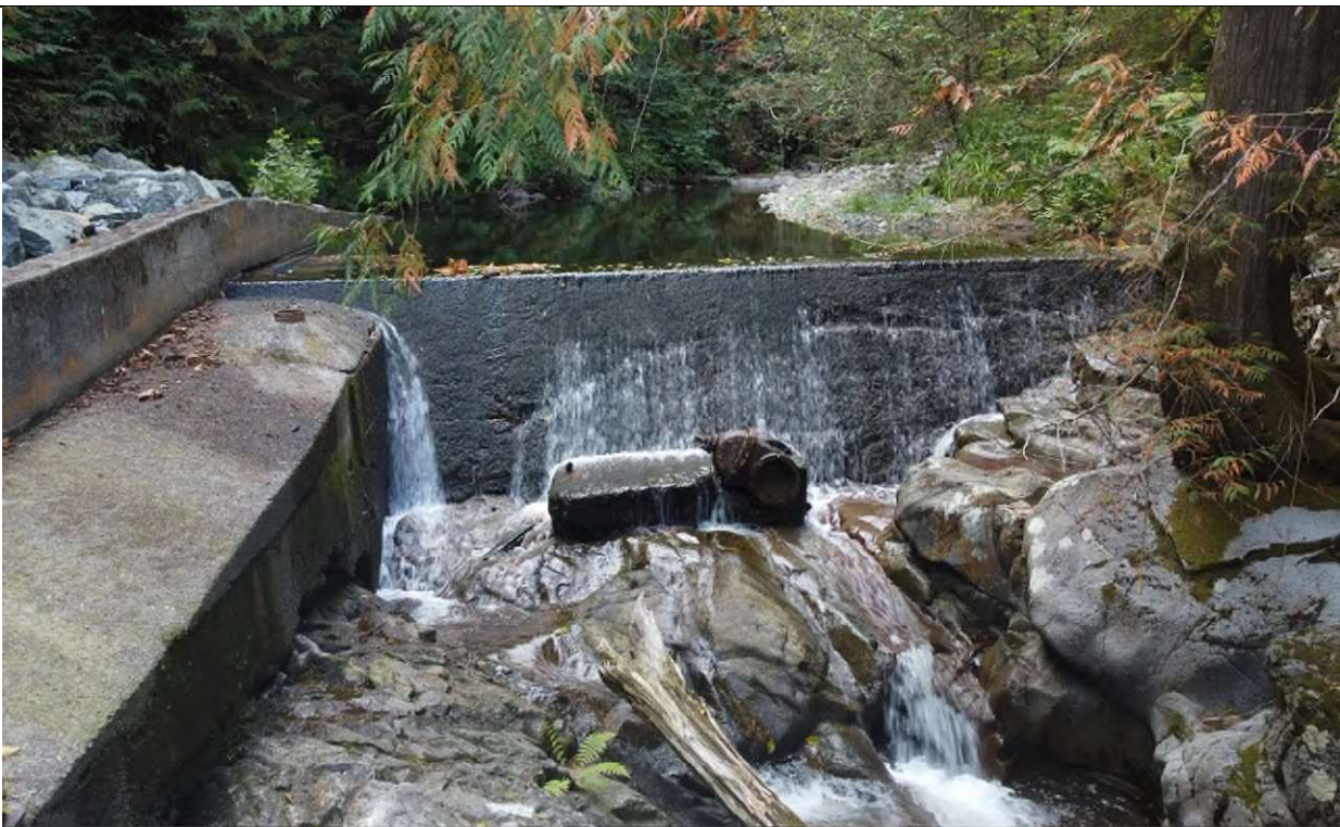
Photo No. 12 Date: 19 September 2023 Looking Towards: West Location: Water Supply Dam Description: Looking at Water Supply Dam during the low flow period.
