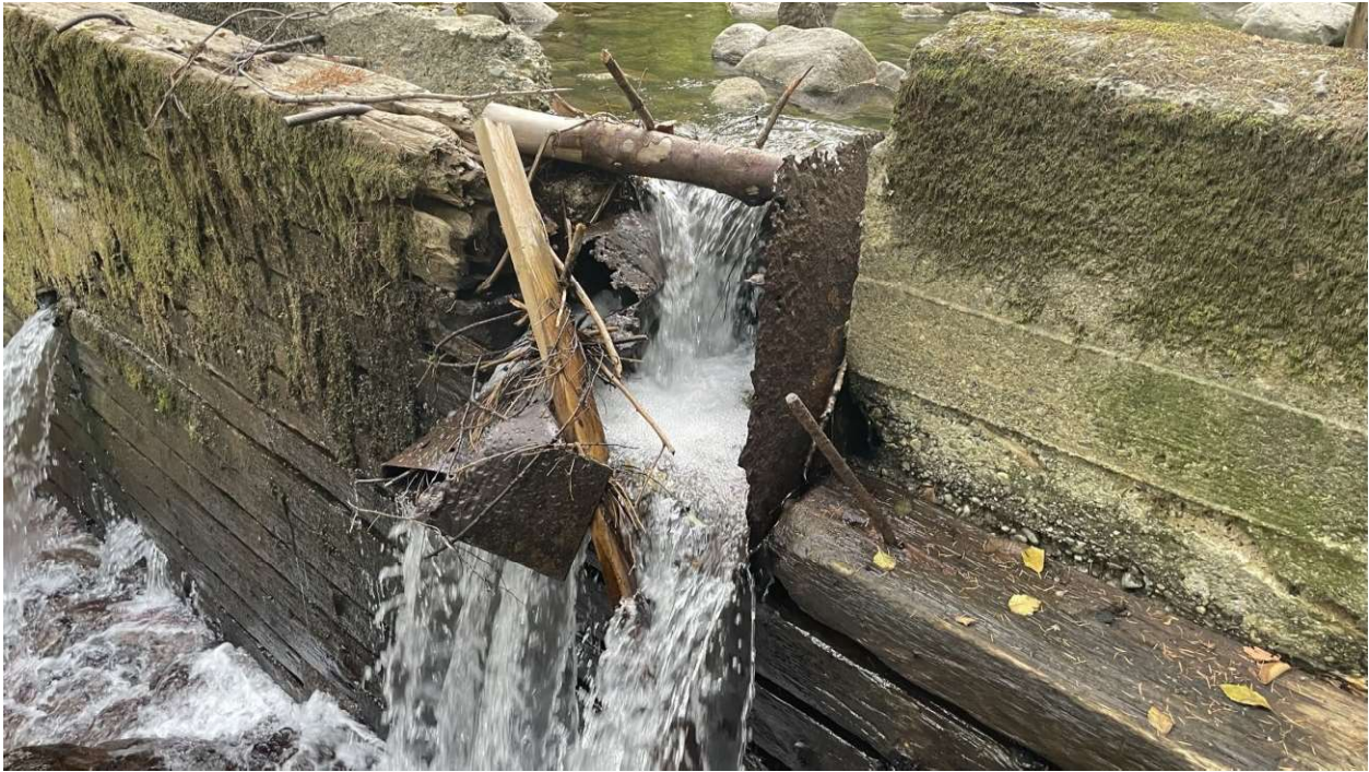
Photo 5 Control Structure on left side, view 2.
