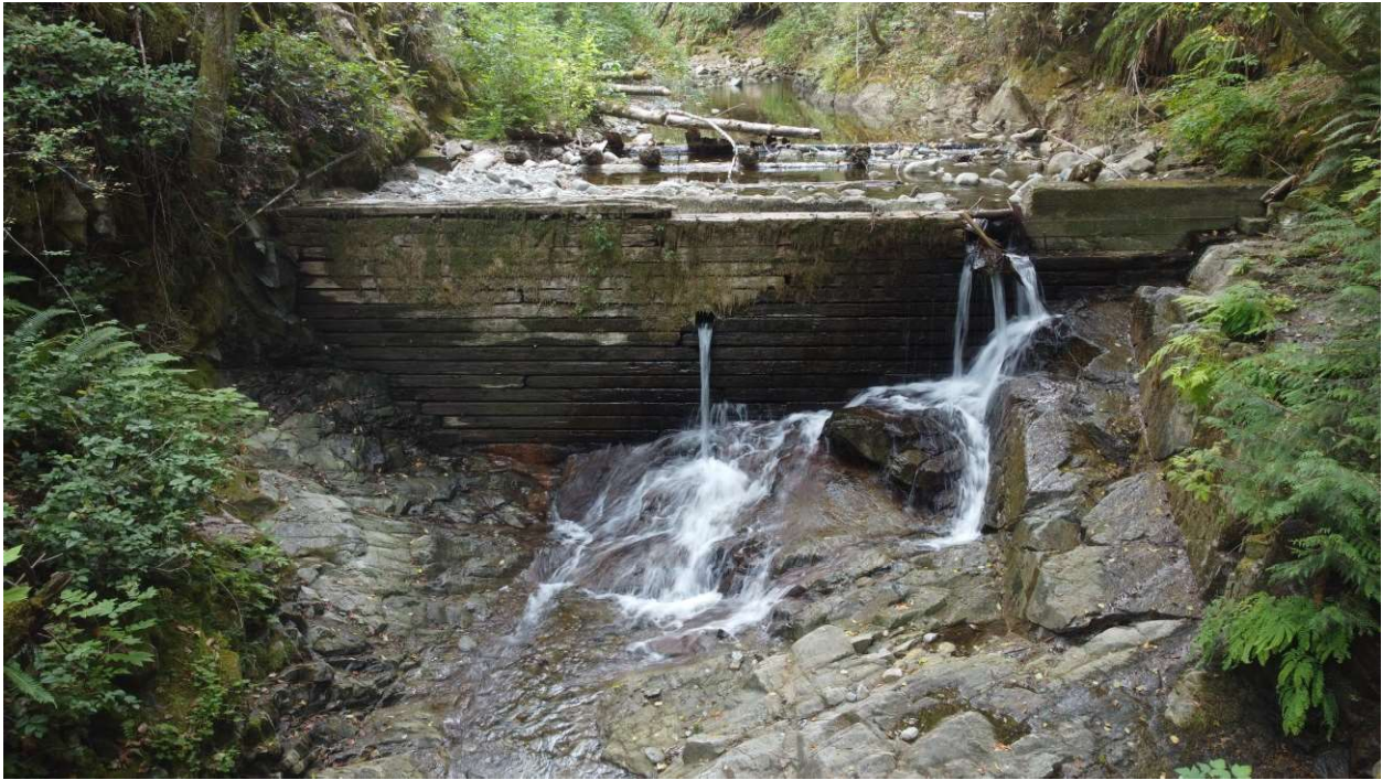
Photo 1 Downstream face of dam, looking southwest.
