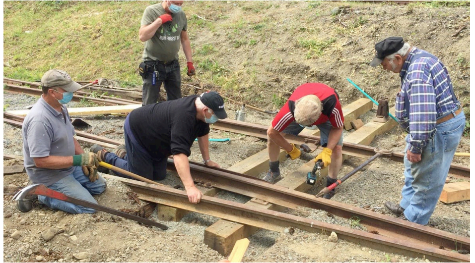
Track restoration / maintenance
