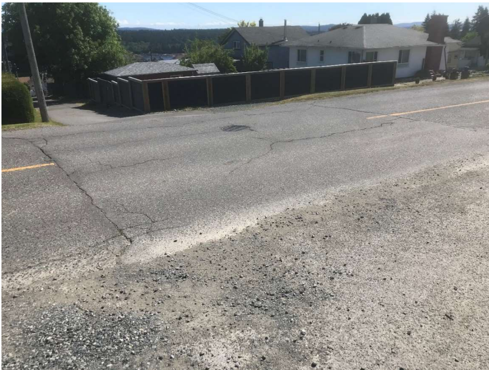
Patch cracking and vertical displacement along major crack lines
