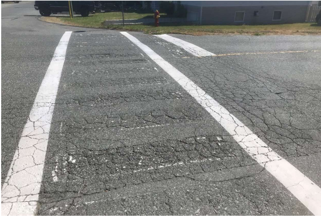
Eradication of road markings causing uneven wear and cracking
