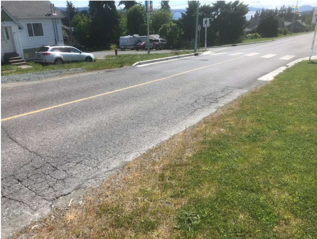
Patch cracking and vertical displacement along major crack lines
