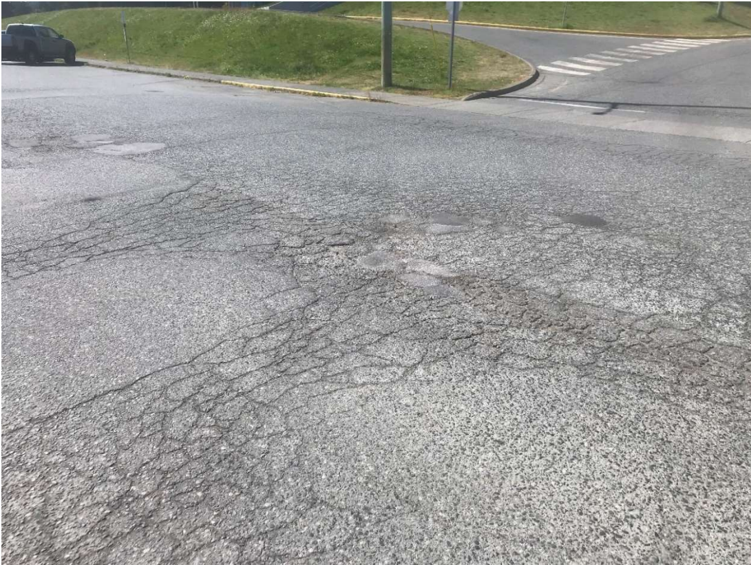
Eradication of road markings causing uneven wear and cracking
