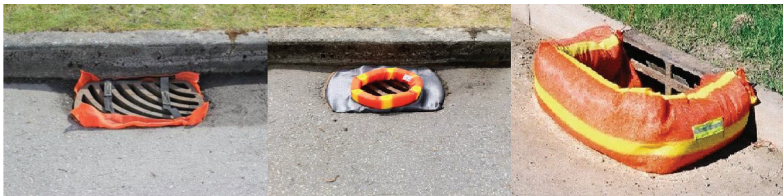
Figure 1. Catch basin inlet protection examples. From left to right: catch basin insert, donut and sediment log.
