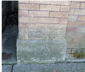
Street level Column with concrete base
