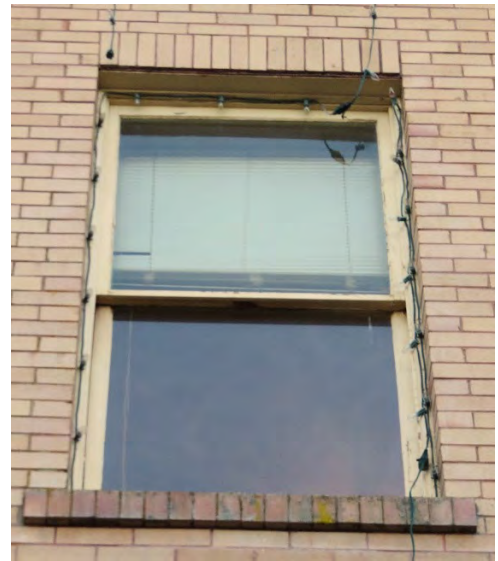
Window brick detailing: Soldier course at head & sill
