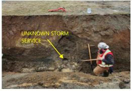
construction process because the storm main was the first piece of work completed. The contractor was authorized to proceed due to the potential flooding risk associated with the small pipe size and to avoid the increased cost of replacing the pipe and service connections at a later date. The cost to complete this work was approximately \$65,000.
