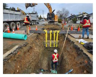
3. The elevation of a proposed watermain was in conflict with an existing BC Hydro duct and it was required to construct the watermain under the duct. This required extensive support of the hydro duct and difficult construction was not originally included.
