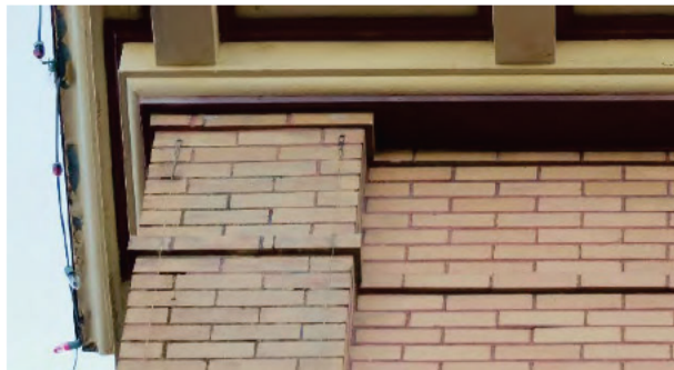
Column expression full height at both corners; two horizontal single brick raised bands;
