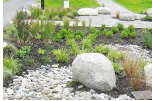
Example of integrated rain water management.
