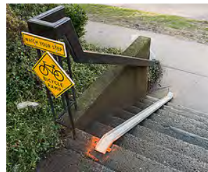
Small scale cycling infrastructure
