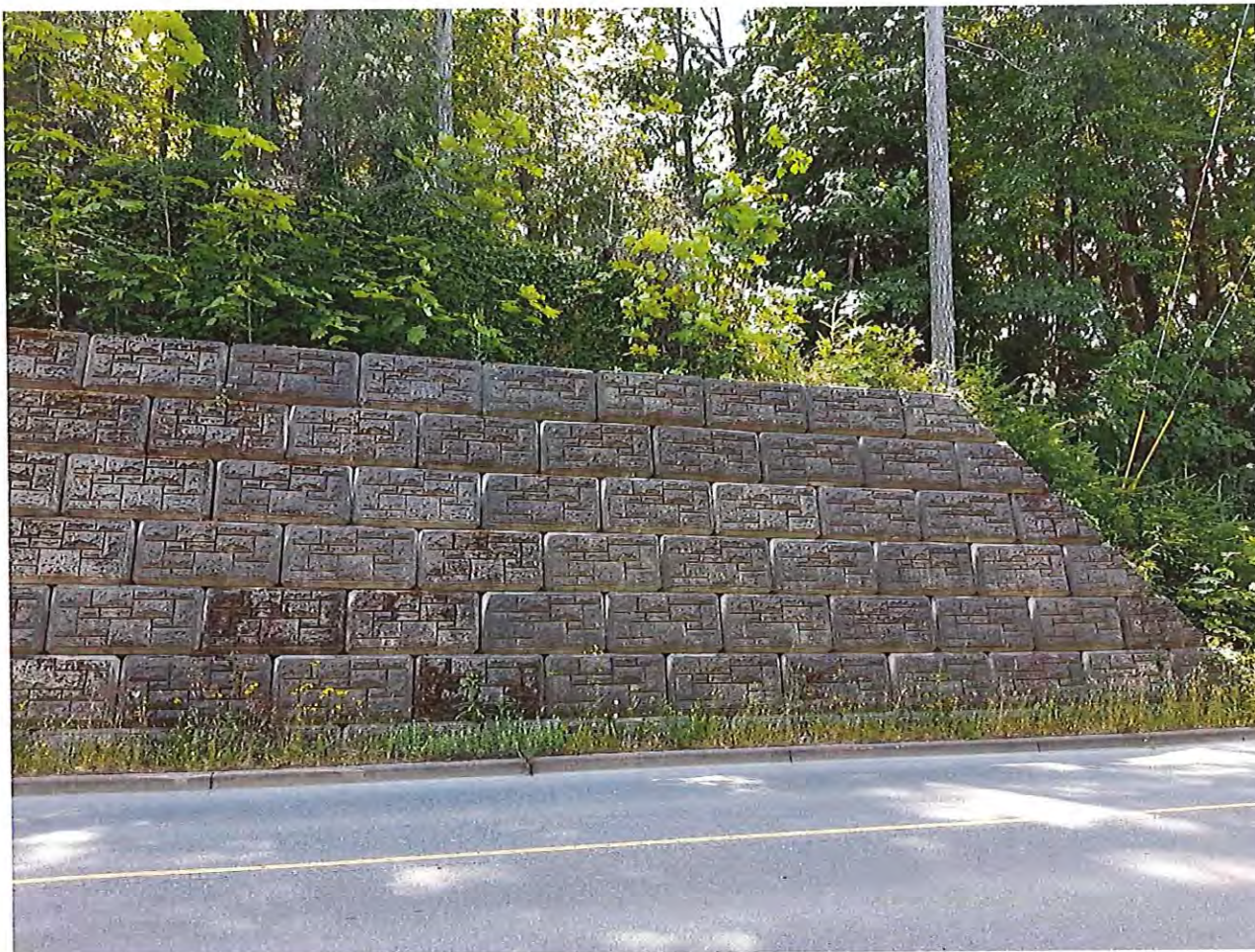
Photo 2.2: Retaining wall near northeast corner of the Property, looking southwest.
