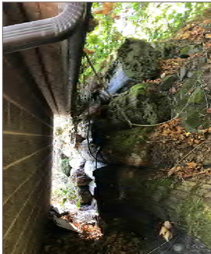
Photo 2: Failing Log Retaining Wall, Looking behind the exiting Power Building
