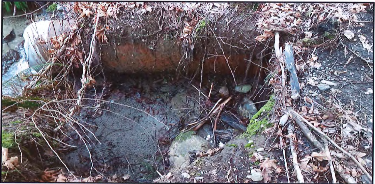
Photo 3: Eroded Culvert
