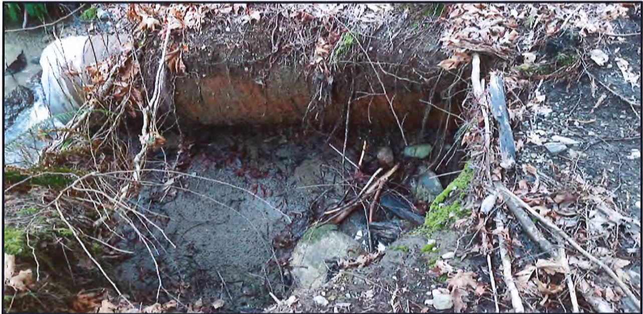
Photo 3: Eroded Culvert
