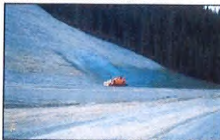
Hydroseeding with mulch, tackifier and grass seed provides a quick cover to exposed soils. Plan work so that seed has time to germinate, and grow before the end of the growing season.
